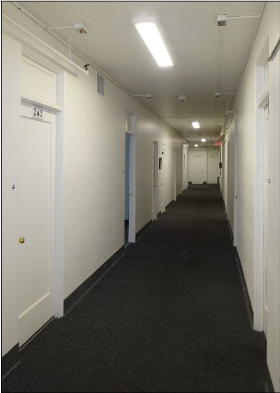
Photo 11 of 14: Second Floor Corridor
