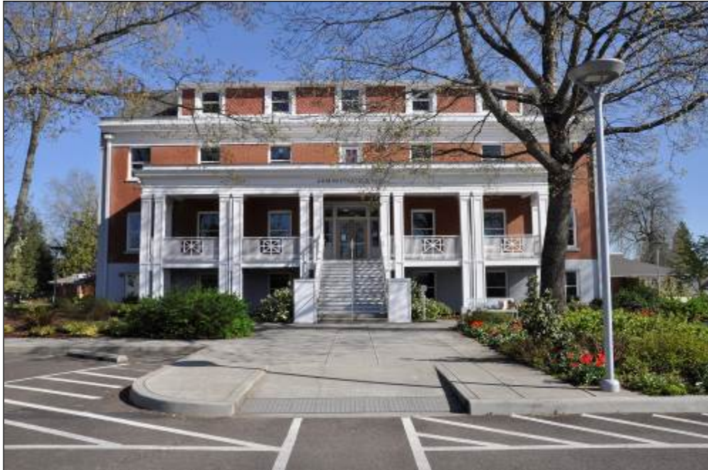
Figure 16: Altenheim Home for the Aged, 7901 SE Division St., Portland.
