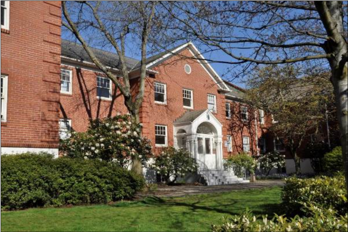
Photo 1 of 14: East elevation.
