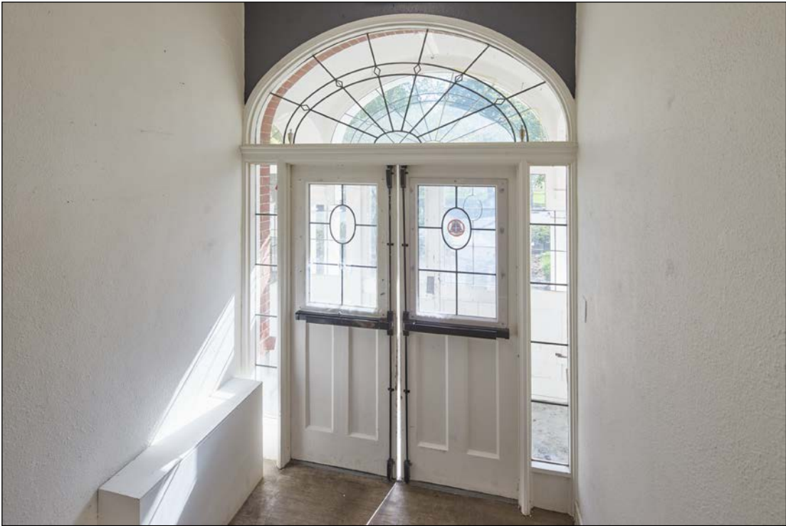
Photo 6 of 14: Main entry.
