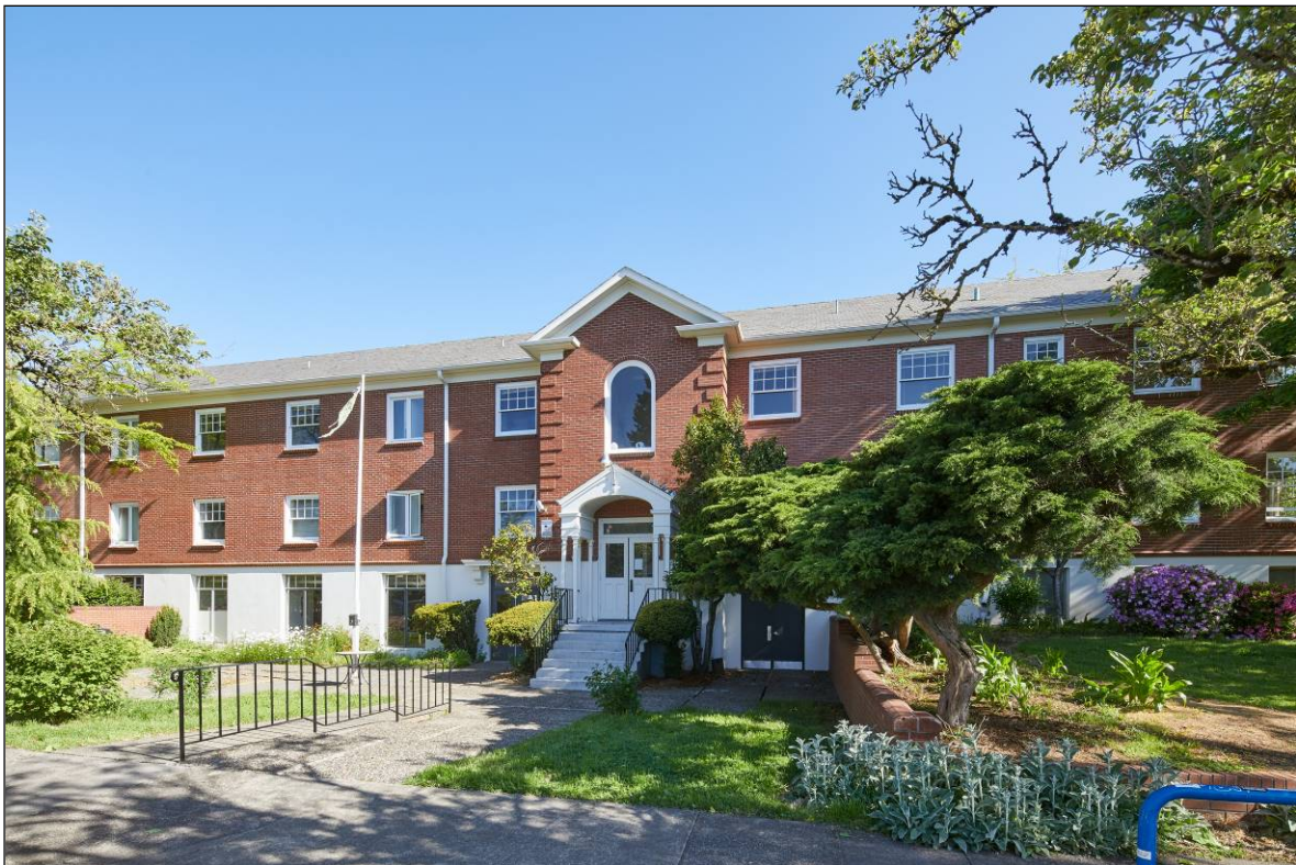
Photo 2 of 14: South Elevation.
