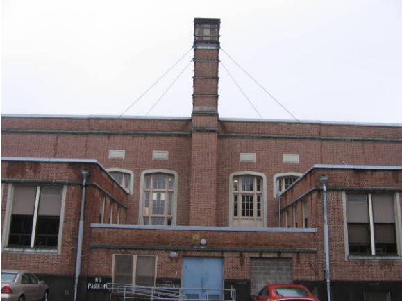
North elevation facing south
