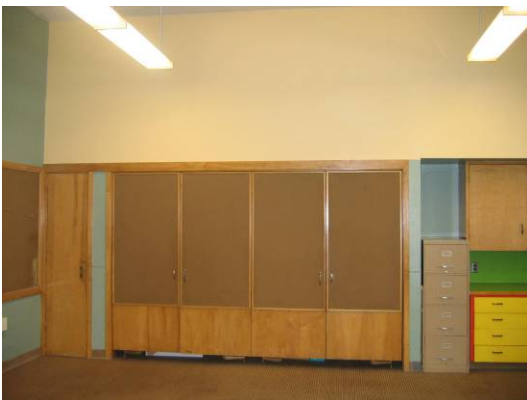
Classroom built-ins in 1950 addition
