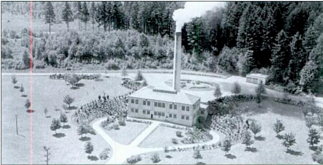
This May 13, 1940, photograph shows the city incinerator, which opened in 1932 on Swift Boulevard, part of today's Columbia Boulevard, and was used until 1970. It was used in conjunction with the St. Johns Landfill located across the street. The facility was converted into the City of Portland's Archives and Records Center in 1981, and the chimney was removed in 1990. (Courtesy City of Portland Archives.)
