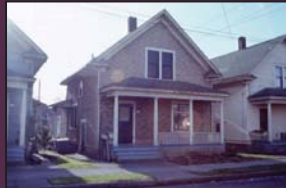
The home of Mrs. Bobbie Verhaegh, 253 N. Ivy St., photographed prior to demolition in 1972. Image courtesy of City of Portland Archive, A2010-003.
