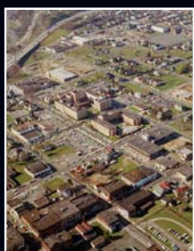
A 1968 aerial of the neighborhood surrounding Emanuel Hospital. Some cleared land can be seen. Image courtesy of Thomas Robinson.
