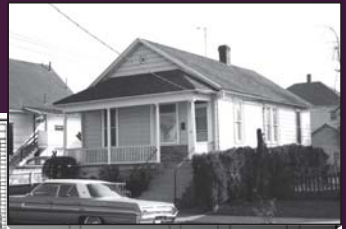
312 N. Cook St., photographed in 1969, was the home of Leo and Ina V. Warren, chairwoman for the Emanuel Displaced Persons Association. It was demolished during urban renewal. Image courtesy of City of Portland Archive, A2010-003.
