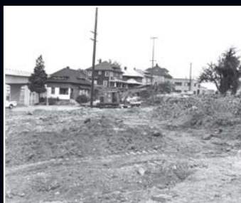
Demolition of properties within the Emanuel Hospital urban renewal project area, September 1972. Image courtesy of City of Portland Archive, A2010-003.
