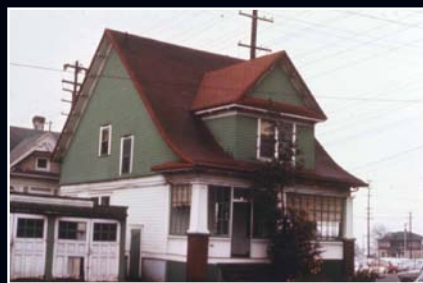
The home of Jake and Bettie Robinson, 122 N. Graham St., photographed in 1971 prior to demolition. Image courtesy of City of Portland Archives, A2000-003.
